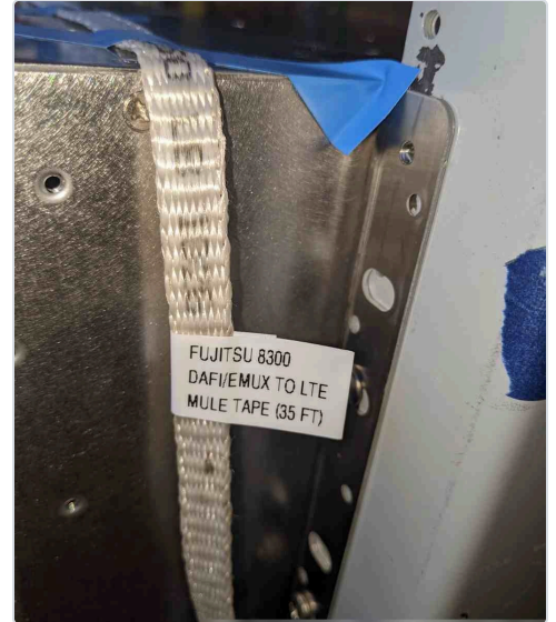
Cable run. Mule tape pull line for a 35 ft cable run, tagged DAFI/EMUX to LTE.
